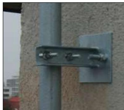
The horn stanchion can be anchored with ropes or can be attached to an inner wall of the building through the roof (see the example pictures)
